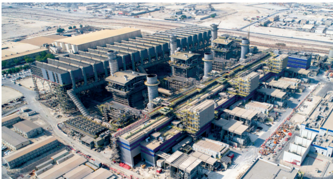
Alba Power Station 5
