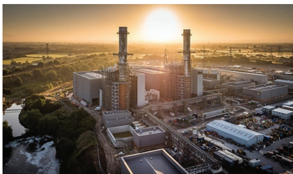
Carrington Power Station (880MW)
