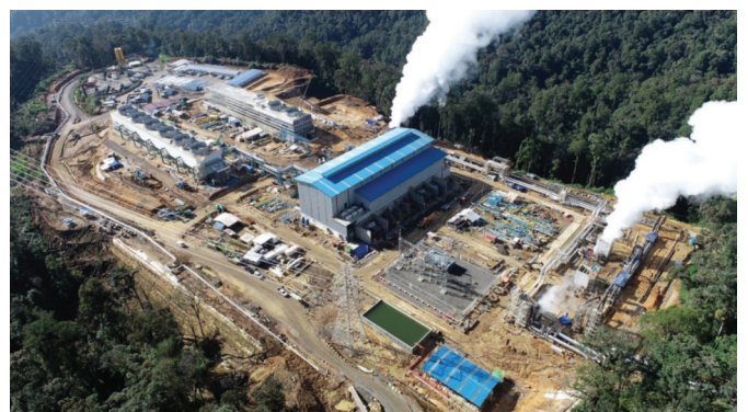
Geothermal power plant on Sumatra
