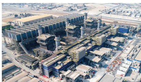
Alba Power Station 5
