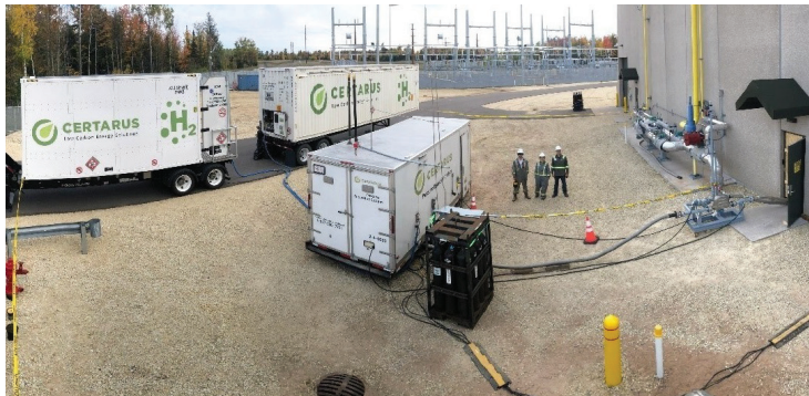
Certarus mobile platform supplies H 2 to the Mihm power station
