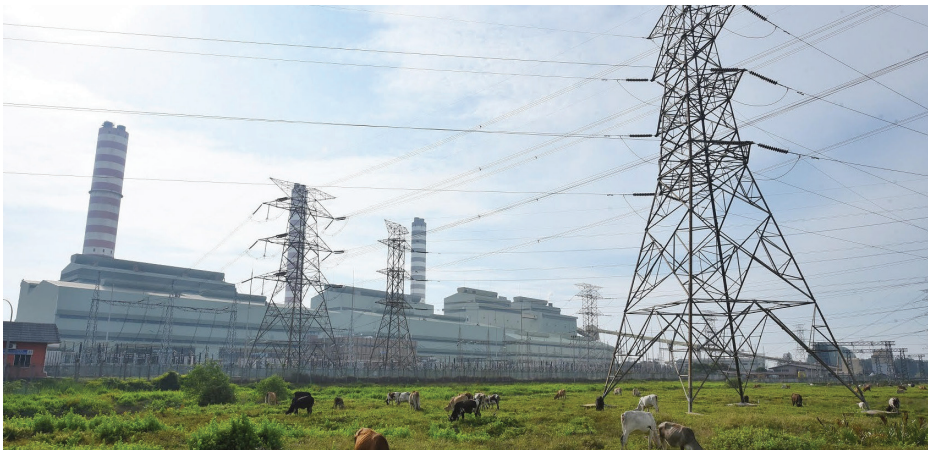
TNB's Abdul Aziz power station near Kapar
