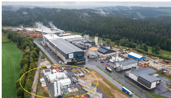
Wunsiedel Energy Park with its new hydrogen plant
