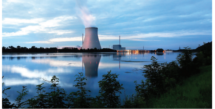
PreussenElektra's Isar-2 plant in Bavaria
