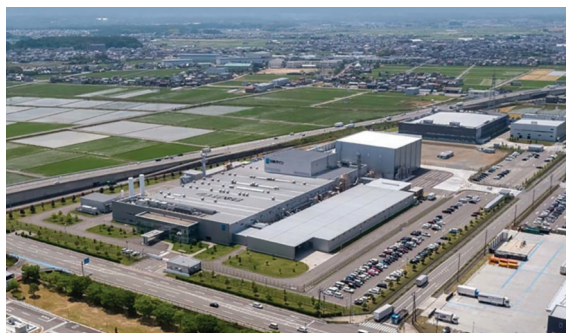
View of NGK Insulators' Ishikawa plant in Nomi City, Japan
