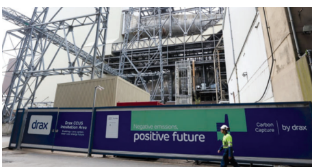
Works have started to retrofit Drax Power Station with CCS
