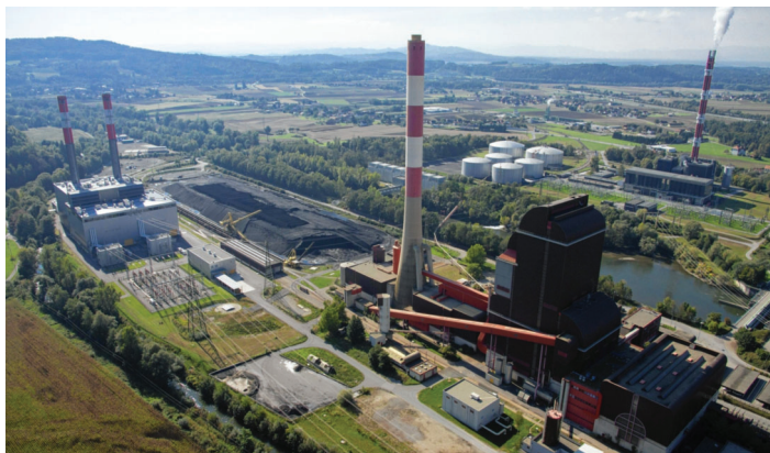
Verbund's Mellach gas power station will be converted to coal
