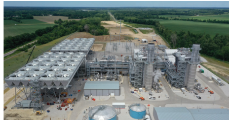
Drone photo of Niles Energy Center
