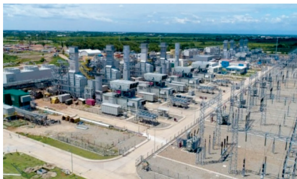
EdM's 450 MW Temane power plant is scheduled to start up in 2024
