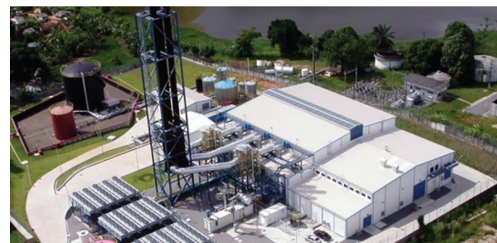
Termocabo gas peaking plant in Cabo de Santo Agostinho
