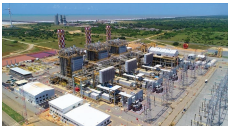
Sergipe Power Plant
