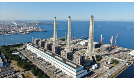
Anegasaki power station in Chiba prefecture
