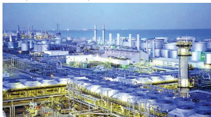
Jazan refinery and IGCC complex
