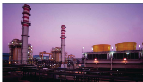
Eni's gas power plant at its Ravenna refinery
