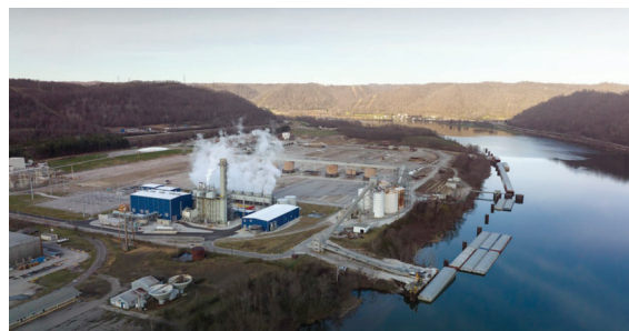
Long Ridge CCGT in Hannibal, Ohio
