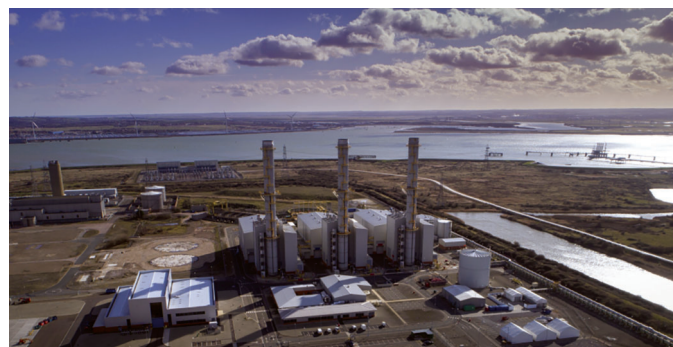
Uniper's H2-ready power station is near the Grain LNG import terminal
