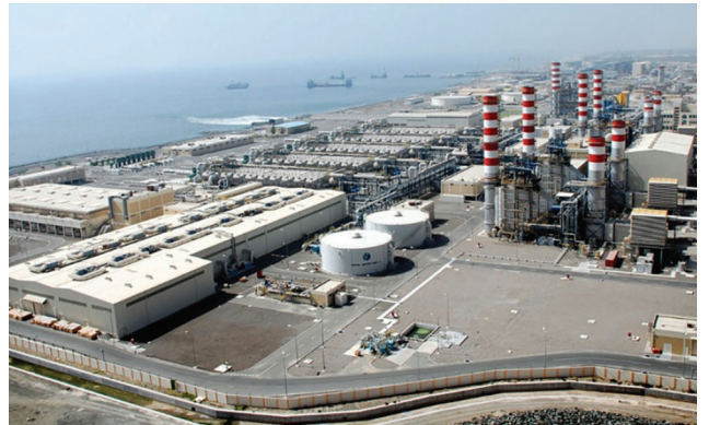
Fujairah F3 is being built between the F1 and F2 units
