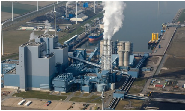
Coal-fired Eemshaven power plant (1.5GW)
