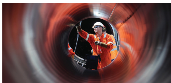
Works on a Nord Stream 2 section near Kingisepp, Leningrad Region
