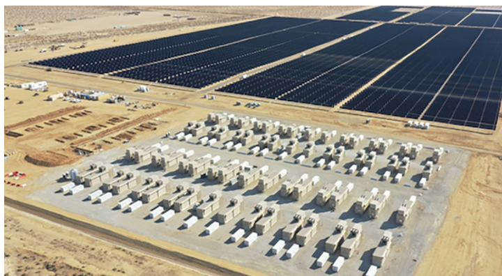
Render of PG&E's Sanborn project Kern County, California
