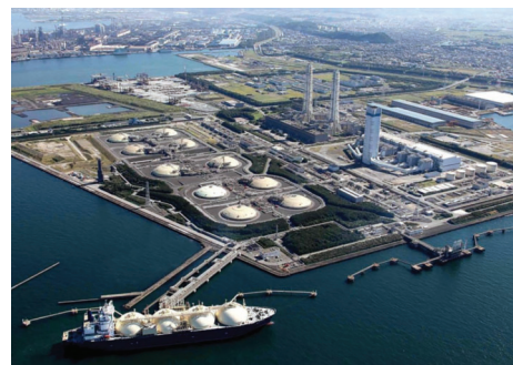
LNG-fuelled power plant in Japan
