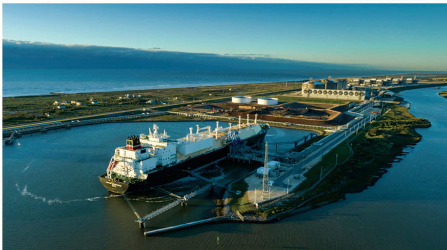
Cargo loading at Freeport LNG on Quintana Island, Texas
