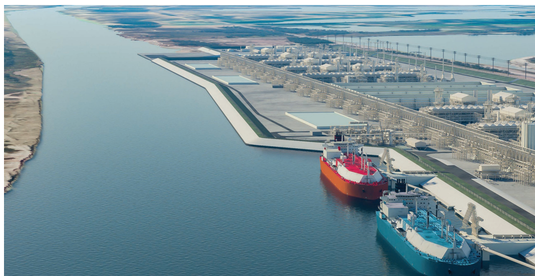
The proposed Rio Grande LNG looking west along the Brownsville Ship Channel
