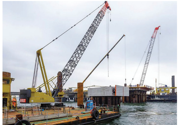
Fenders were installed at Wilhelmshaven's first LNG terminal ready for the opening
