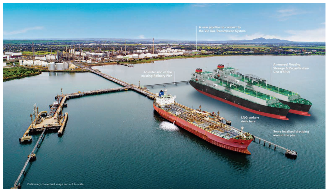
Woodside is set to join the consortium to develop the Geelong regas terminal
