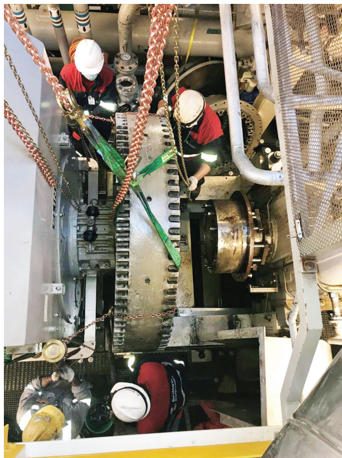
Burckhardt's team seen working on the compressor skid in the confines of the compressor machinery room (CMR)
