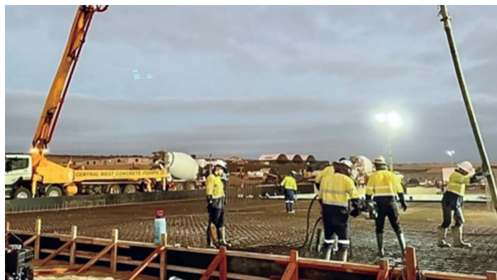
A Clough team working on part of the Waitsia gas and LNG project near the town of Dongara, about 350km (217 miles) north of Perth and 65km south of Geraldton
