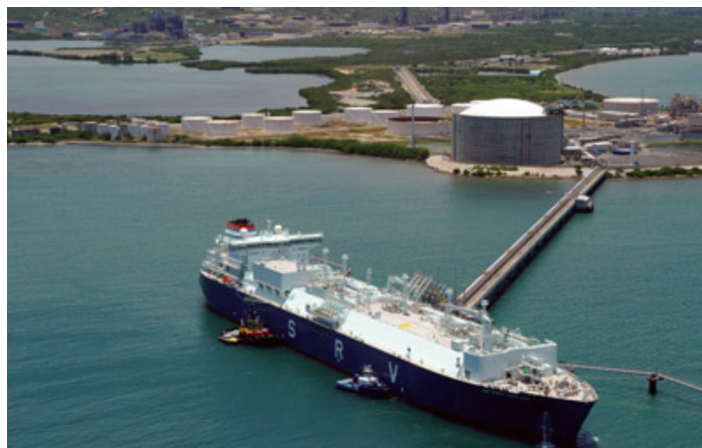
Peñuelas terminal in Puerto Rico operated by EcoEléctrica
