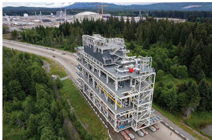
A giant module for liquefaction plant is delivered to site
