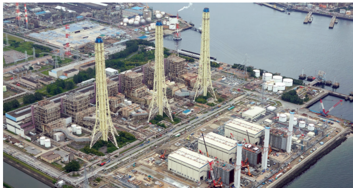
Anegasaki power station uses regasified LNG deliveries
