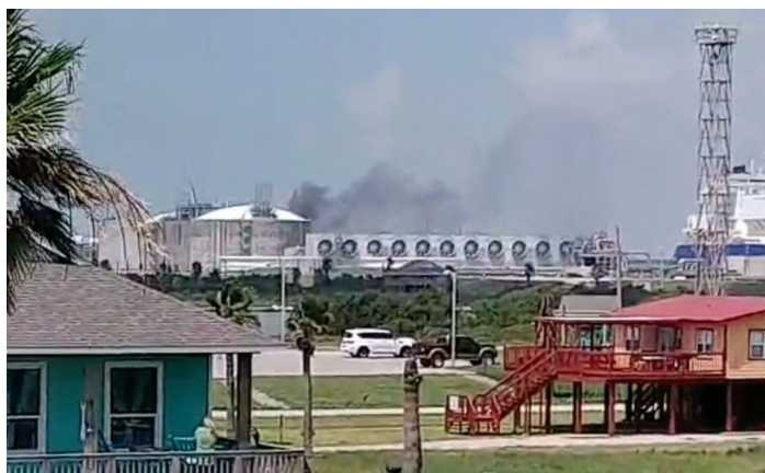
Smoke billows from Freeport plant after the June 8 explosion
