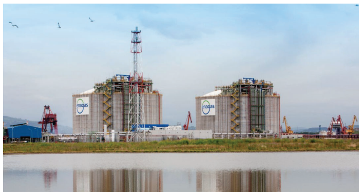
SNAM and Enagás could combine eight LNG terminals
