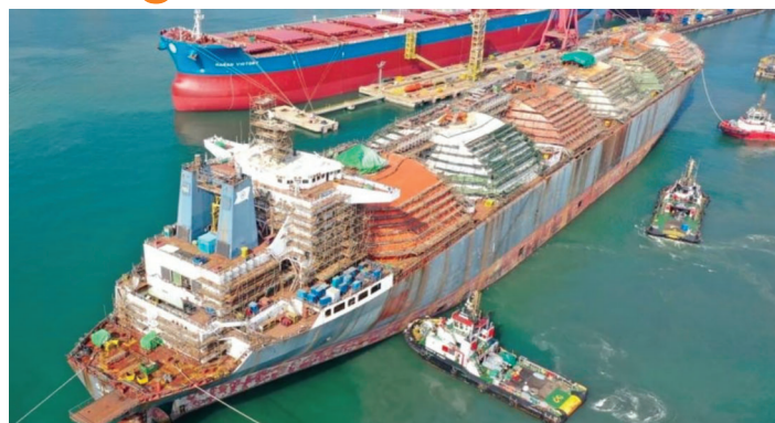
Carrier 'Gimi' being converted to FLNG hull in Singapore
