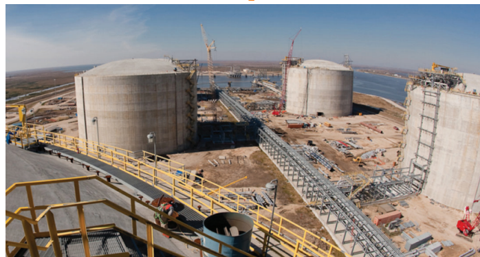
Golden Pass is on the Sabine-Neches Waterway in Texas
