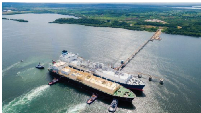
Vopak's LNG Terminal in Colombia has capacity of 4 Bcm
