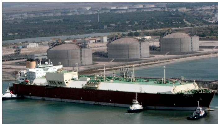
French Fos Cavaou LNG terminal sited west of Marseille
