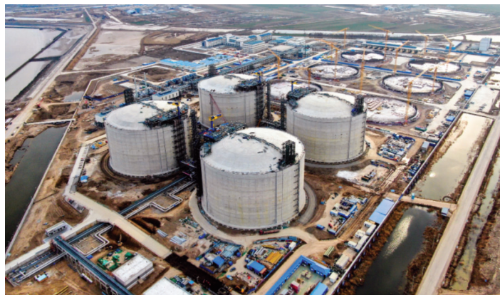
Total of 10 LNG tanks are being built with four completed
