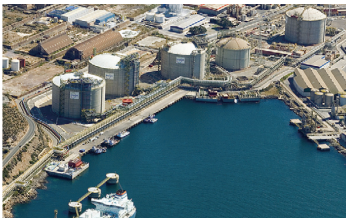
Cartagena import terminal in southeast Spain has five storage tanks and three bays for truck loading
