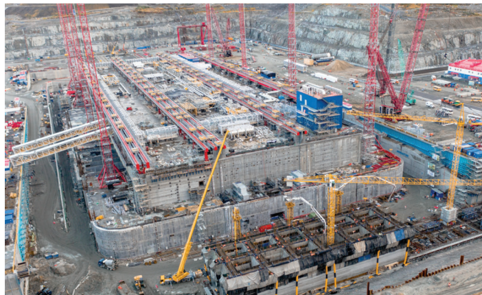
Arctic LNG II's gravity-based plant is being built at Novatek's yard at Belokamenka in Murmansk Region
