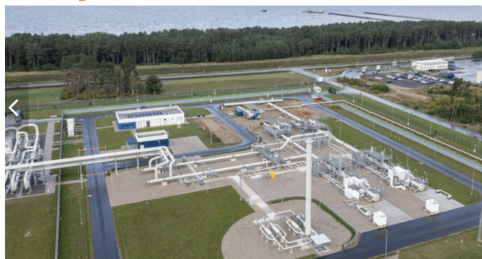
Landfall at Lubmin in Germany for new Russian pipeline
