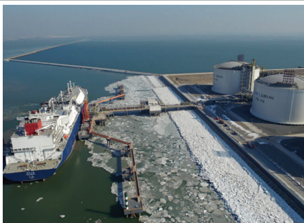
LNG carrier berthing at Tianjin regas terminal, operated by Sinopec
