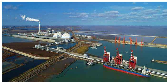
Binhai Port, where CNOOC builds new LNG storage tanks
