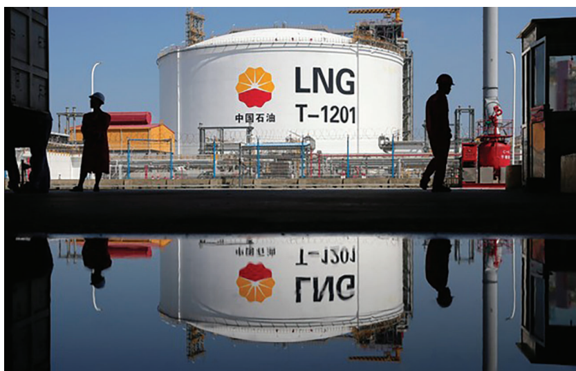
Workers in front of PetroChina LNG storage tank
