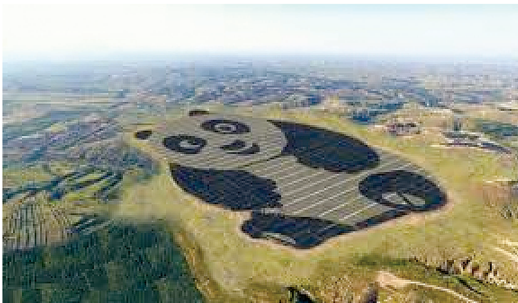
Panda-shaped 50 MW solar PV project in Datong, China, built by UNDP and Panda Green Energy.
