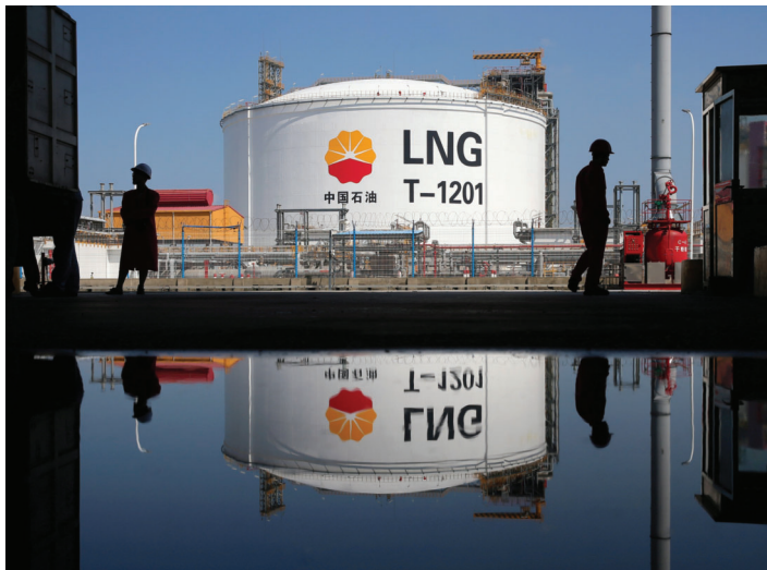
Workers in front of a PetroChina LNG storage tank
