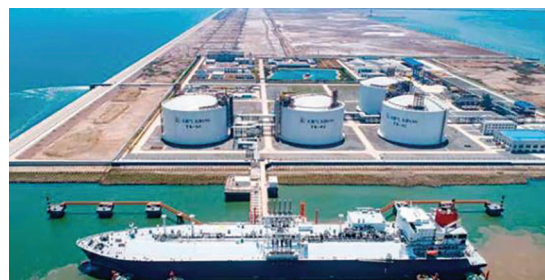
Sinopec is building five new storage tanks at its Tianjin LNG terminal
