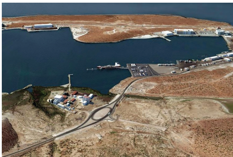
Site of Pichilingue LNG, under construction north of La Paz
