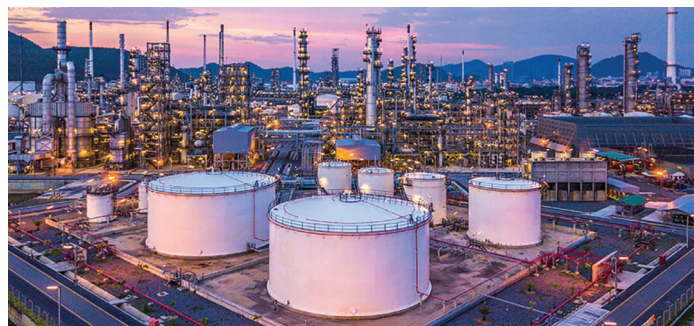
Waha Gas Storage will be connected to the Agua Blanca and Whistler pipelines
