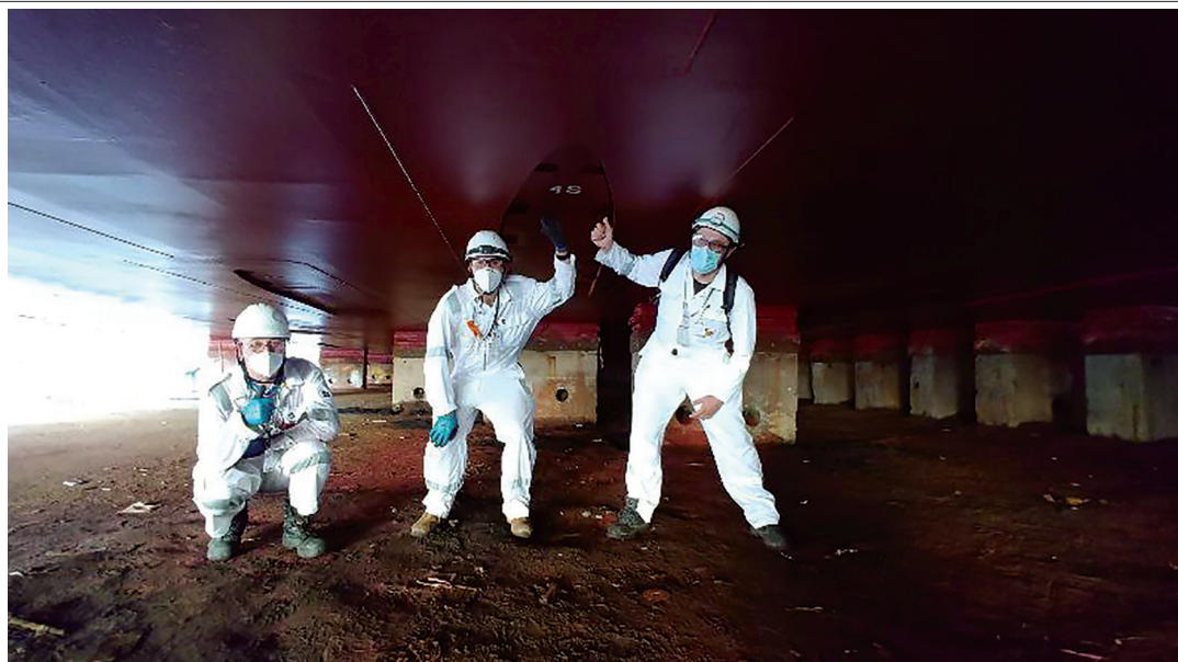
The LNGCs underside with the air lubrication system
