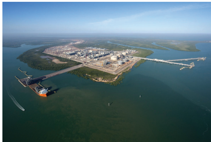
Ichthys shown while under construction
