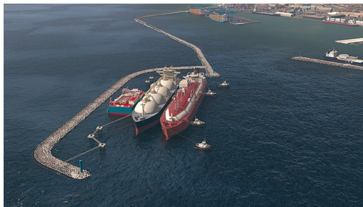
Consultancy work has concluded on the Tema LNG project
