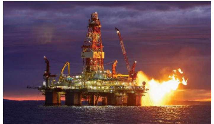
Cooper Energy's Sole gas field in the Gippsland Basin
