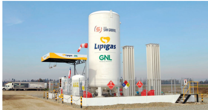
Chilean LNG fuel facility is close to Pan-American Highway
