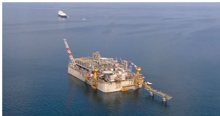
Terminal has been on line since 2009 and is 17km offshore
