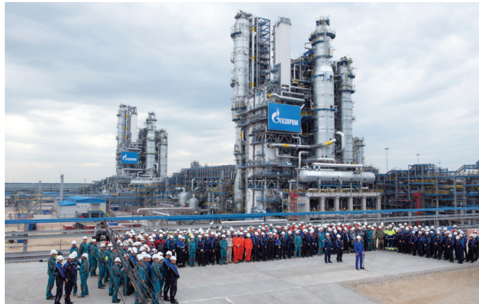
There were virtual and on-site events to start plant
