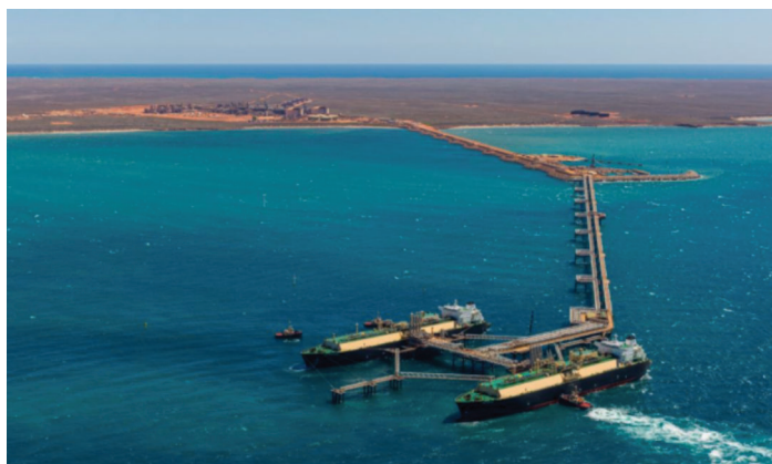
Gorgon plant loading on Barrow Island in Western Australia
