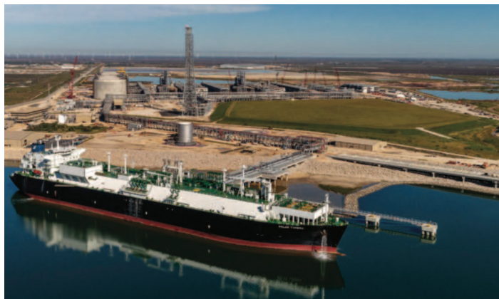
US Corpus Christi plant to be expanded (Photo Bechtel)
